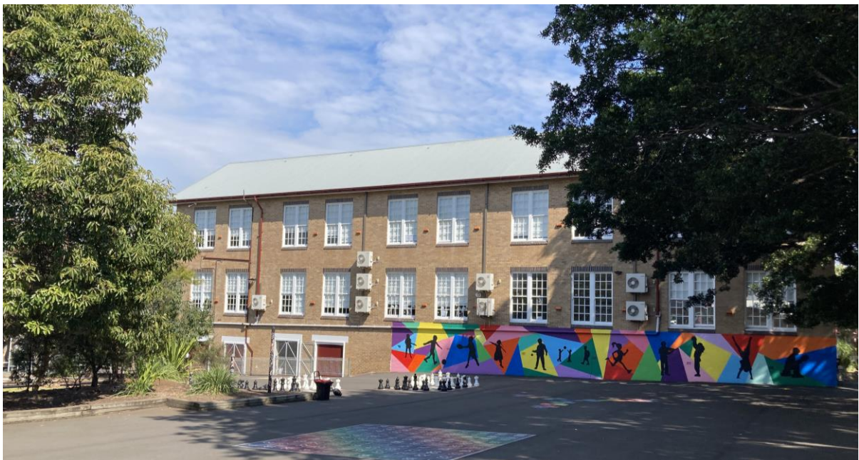
Figure 15: Eastern elevation of Block A building (item 3614).
