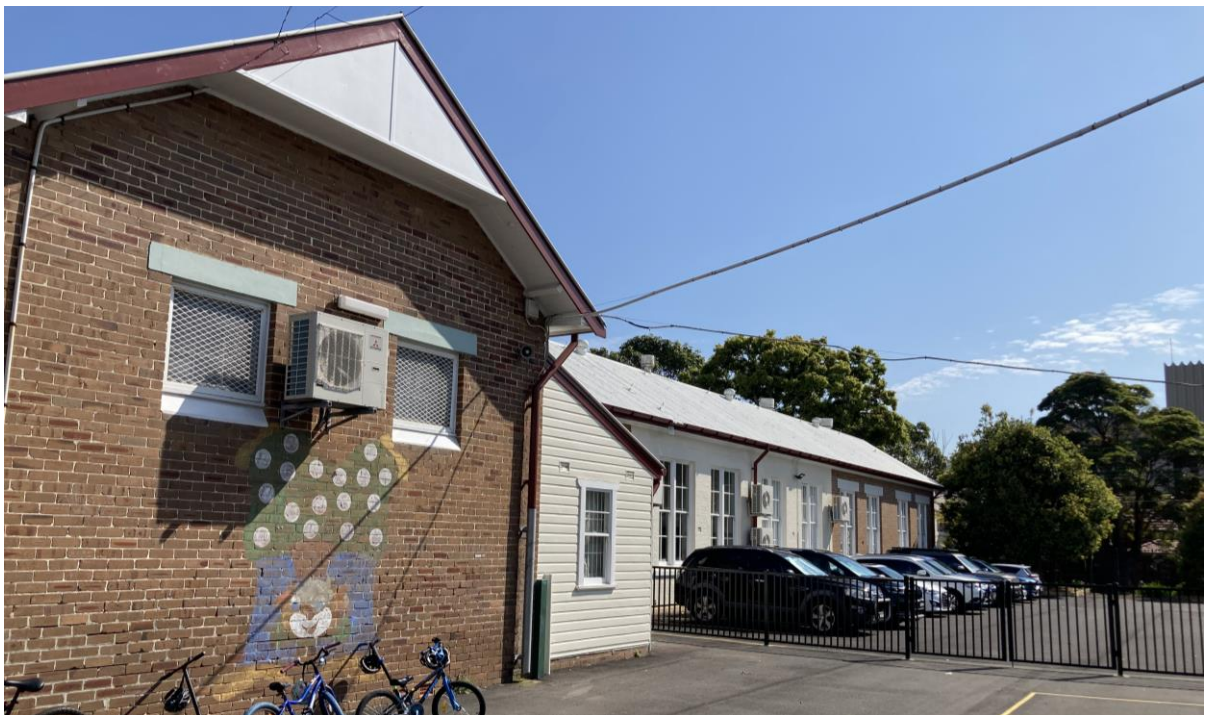
Figure 17: Eastern elevation of Block B (item 3618).
