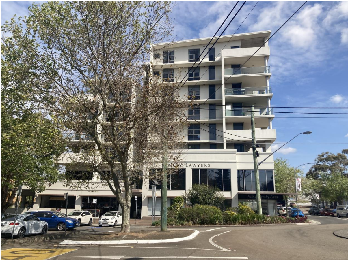
Figure 9: View at intersection of President Avenue and Merton Street facing west, showing multi-storey mixed development.
