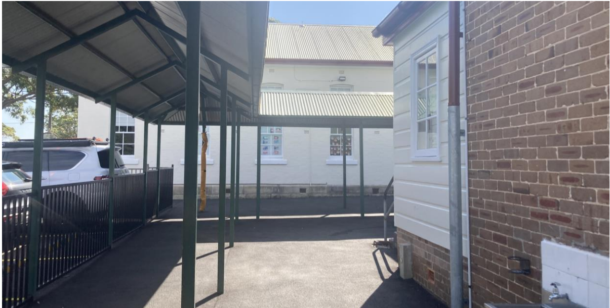
Figure 18: View of painted brick elevation of Block A building, near staff carpark (north-western corner of school).
