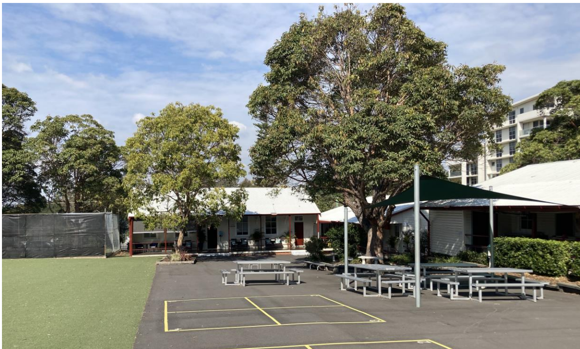
Figure 25: View facing south of Blocks G, H and I on the south-western corner of the school.
