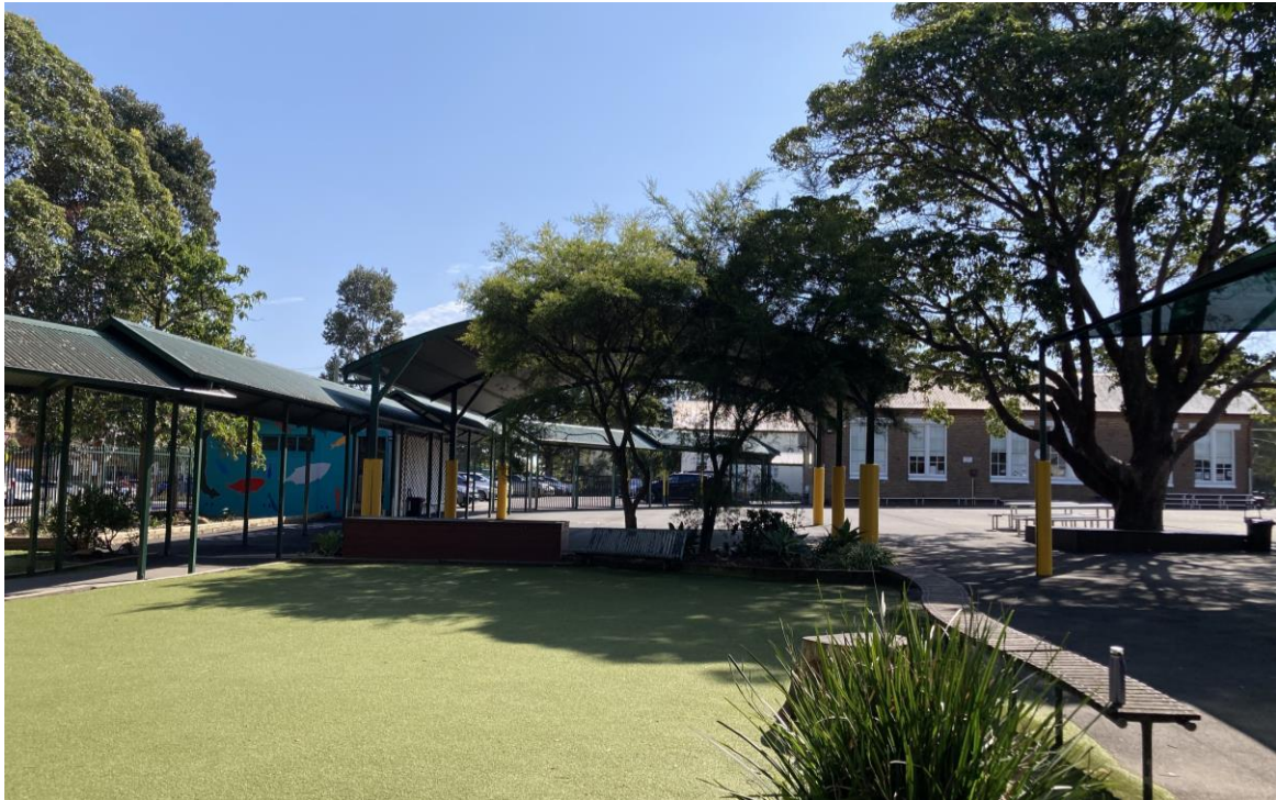
Figure 26: View facing north from Block A (item 3618) of the covered walkway, covered paved area and canteen building (Block J), where the medium hall with canteen is proposed to be constructed.
