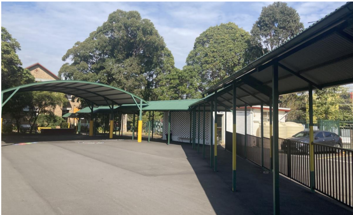
Figure 27: View of covered walkway, covered paved area, Block J and edge of staff carpark, where the new medium hall with canteen is proposed to be situated.
