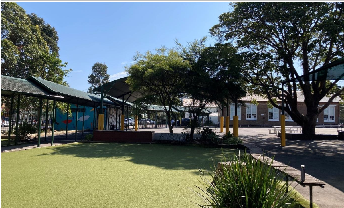
Figure 49: View from ground floor of Building A looking towards Building B (background), which is obstructed by trees, covered walkways and the Cola.
