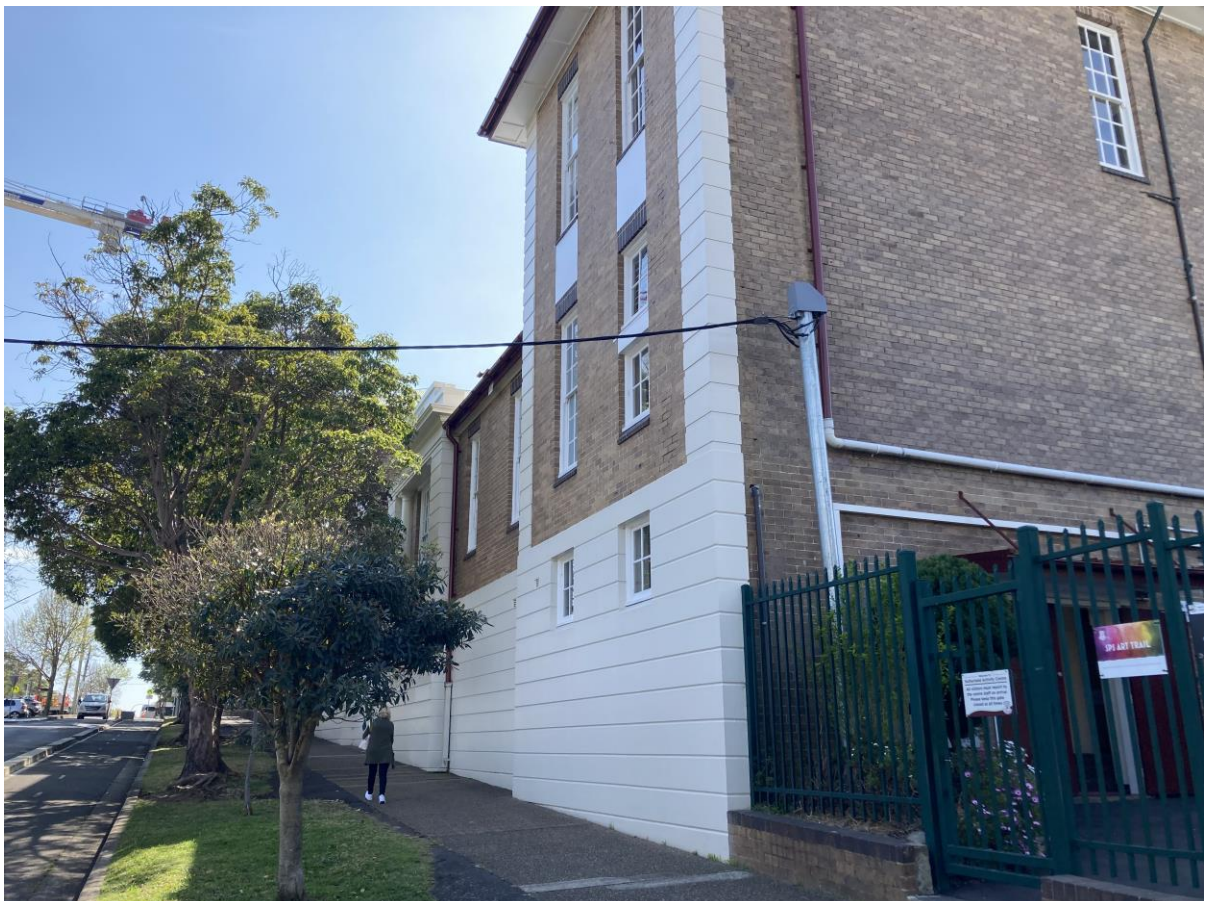
Figure 13: Western elevation of Block A building (item 3614).
