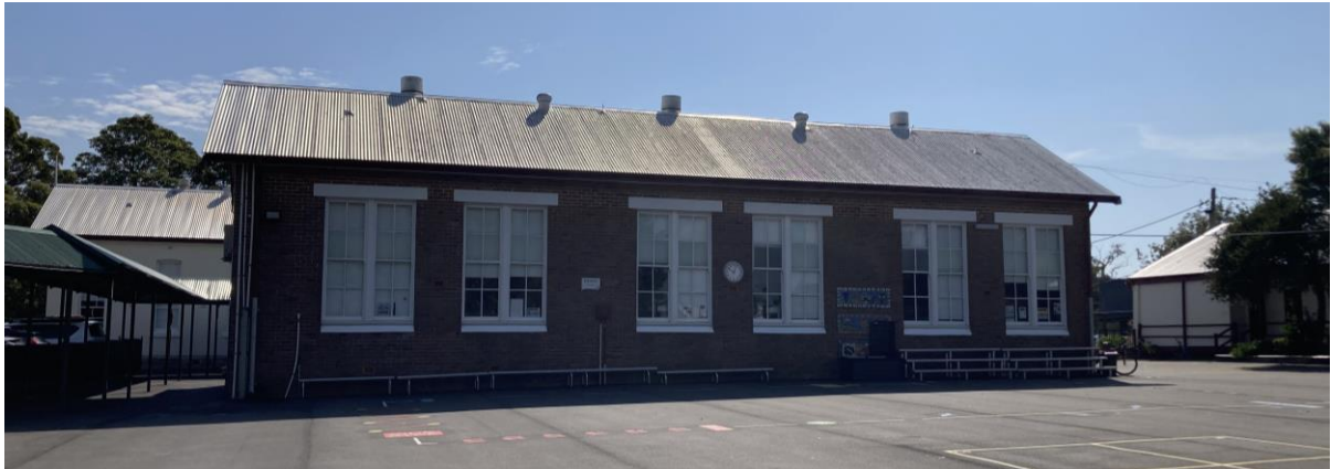
Figure 16: Southern elevation of Block B building (heritage item 3618).
