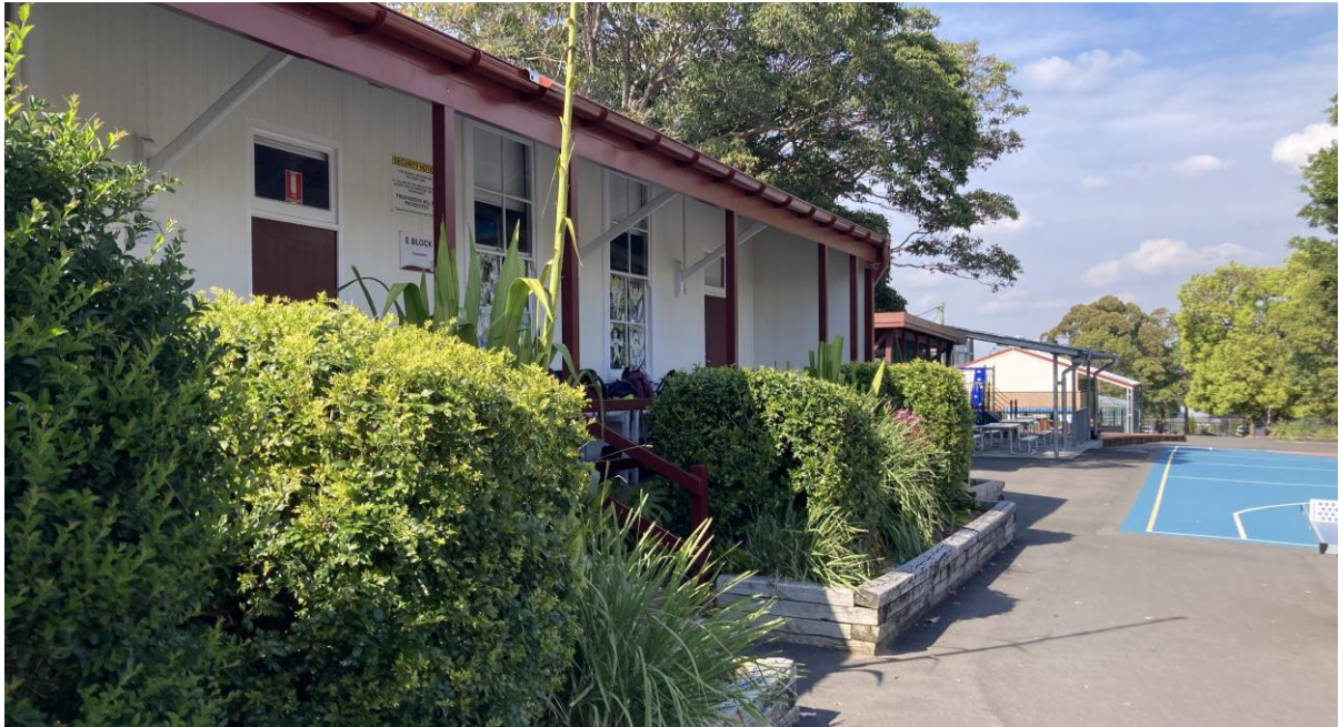
Figure 22: View of original features of the Block E building including single hung timber windows and timber brackets.
