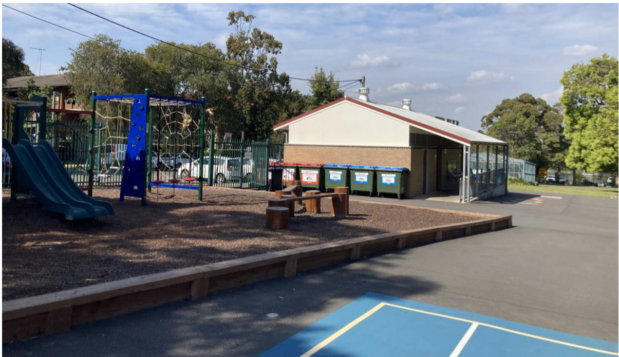
Figure 23: View of Block K toilet block and playground equipment on Merton Street boundary.
