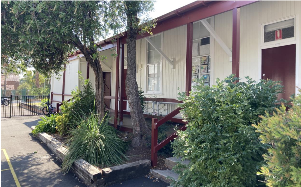
Figure 20: View of original features of Block D building, including single hung timber windows (with glazed panes) and timber brackets.
